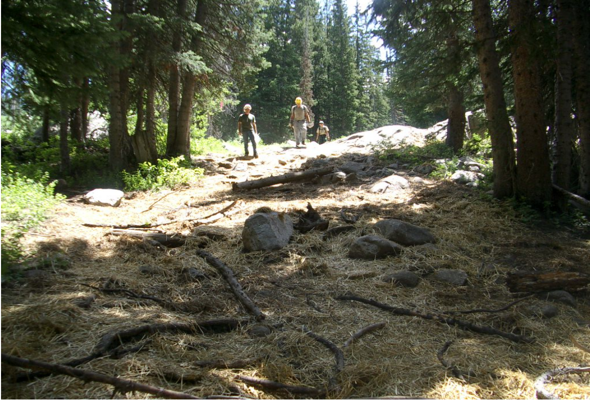
The same location after being reseeded with native grasses and covered with weed-free straw.
