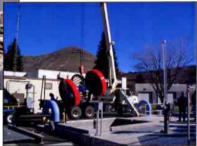
Crane lifting "pig" into "pig" launching structure at Deer Creek Dam.
