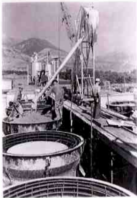
A-40-69 Pouring concrete for 69 inch diameter precast concrete pipe. 7-19-69--Bur. of Reclamation photo., W. S. B.
