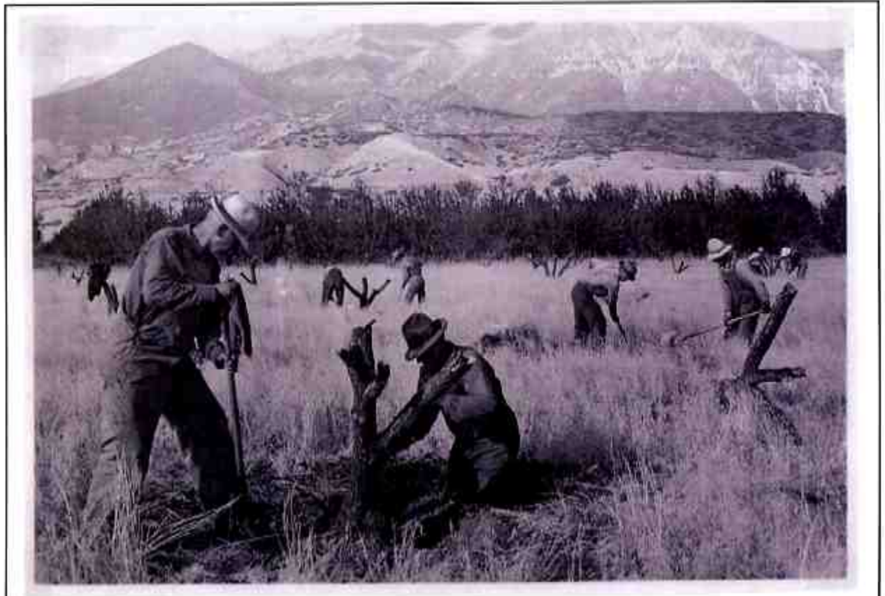
PR-425 Deer Creek and Salt Lake Aqueduct Divisions. An inadequate water supply was disastrous to a portion of this orchard. Water from Deer Creek Reservoir on the Provo River Project will alleviate future losses. 9-12-40--Bur. of Reclamation photo., J. C. Allen.
