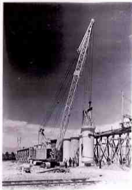
A-50-78 Pipe Line. Lowering pipe to plant pond. 5-2-69--Bur. of Reclamation photo., W. S. B.
