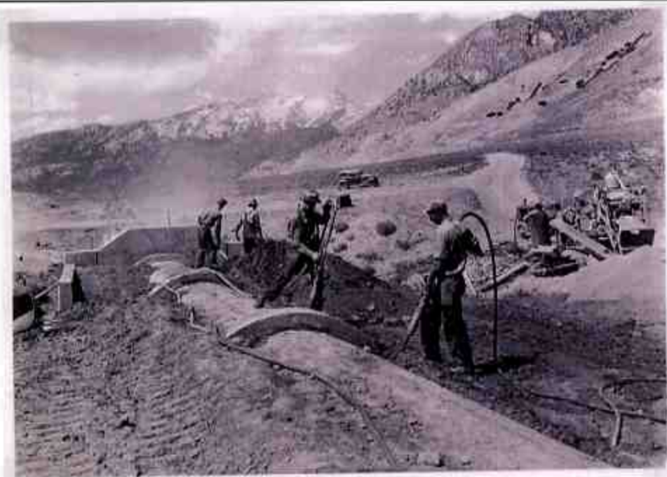
PR-389 Deer Creek and Salt Lake Aqueduct Divisions. Hand tamping backfill around pipe and drainage span structure near Station 998, Salt Lake Aqueduct. 8-9-40--Bur. of Reclamation photo., J. C. Allen.
