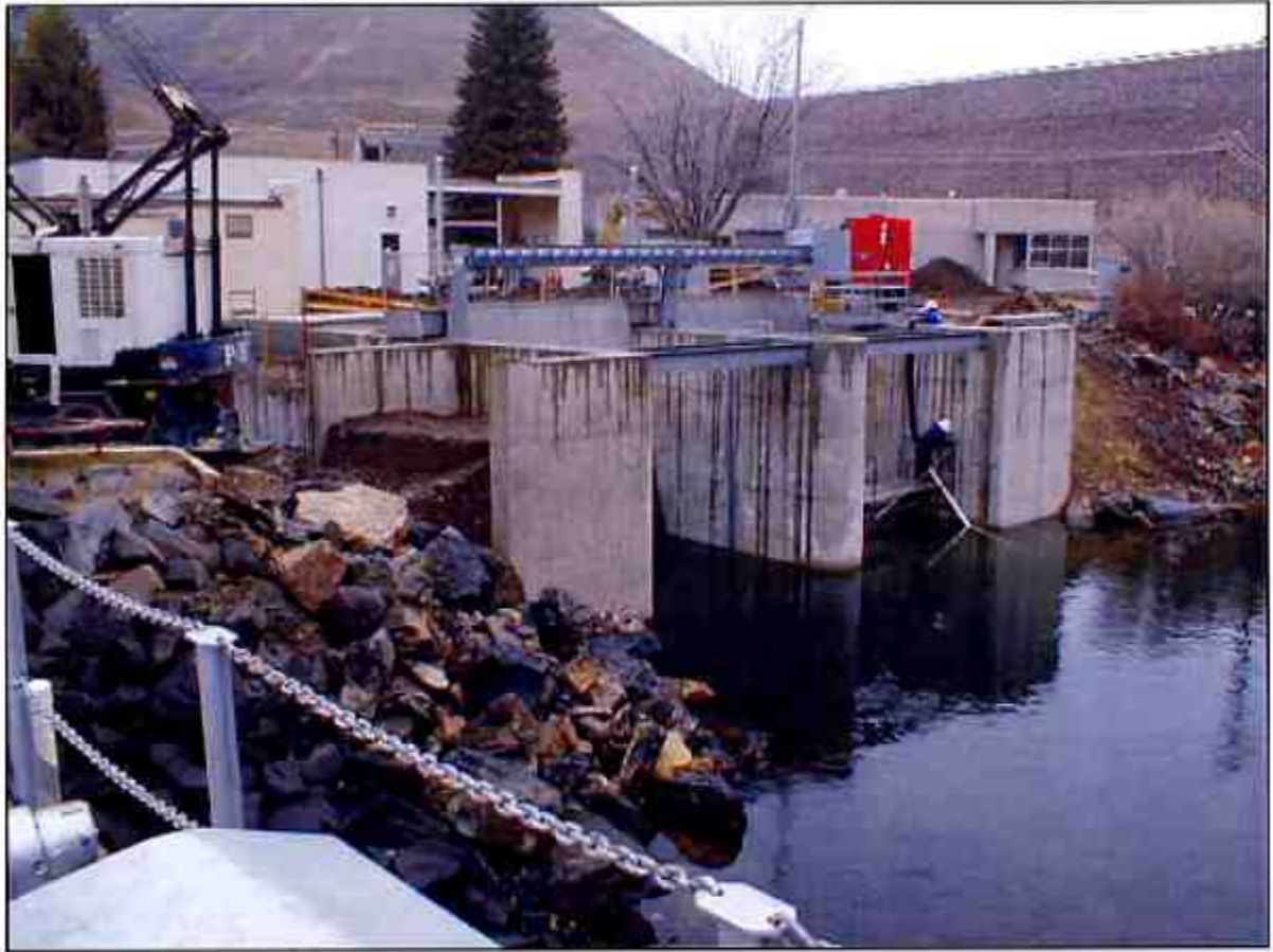
Salt Lake Aqueduct Intake at Deer Creek Dam.
