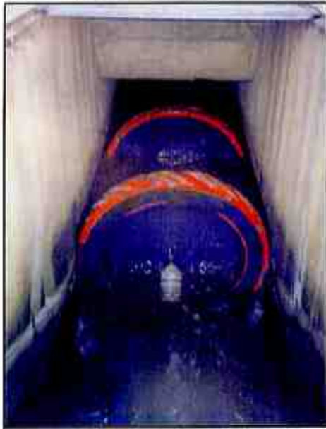
"Pig" entering the Salt Lake Aqueduct
