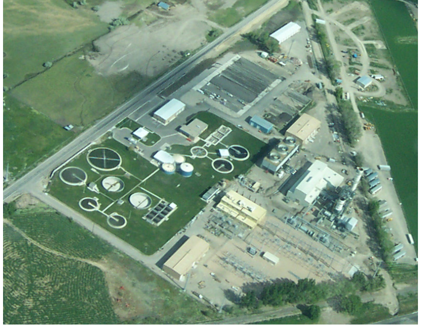
The Nebo Generating Facility is located adjacent to Payson City's Wastewater Treatment Facility to take advantage of the available reclaimed water for cooling tower purposes. (Photo courtesy of Utah Association of Municipal Power Systems.)
