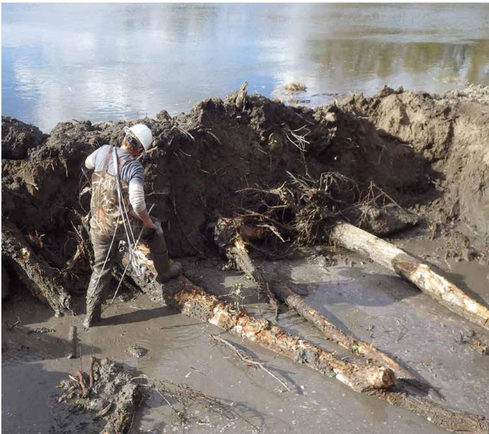
County Watershed crew member standing on the lower trunk of a toe-wood structure (closest to the root wad) to stabilize the trunk during installation.
