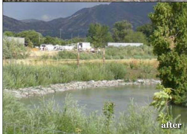
*Vertically eroding banks are clearly visible in the “before” picture at one of seven Jordan River sites to receive stimulus funds for restoration. Bank stabilization included regrading the banks, placing a rock layer to protect the base (toe) of the slope, and revegetating with native plants.*
