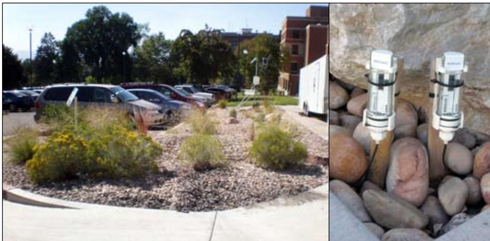
*What looks like a typical commercial landscape is actually a bioretention garden that collects and uses stormwater runoff at the University of Utah's Civil & Material Engineering building. Soil moisture meters (right) are used to monitor effectiveness, with the goal of installing bioretention gardens campus-wide.*
