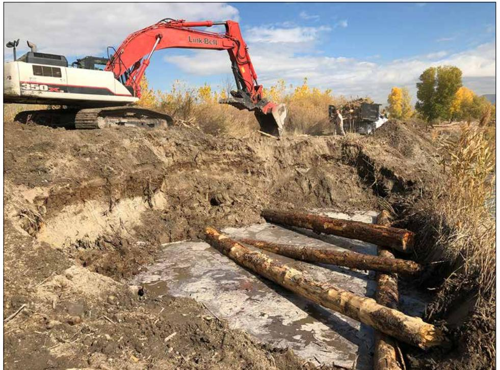
Over 150 logs were used to build the toe-wood structures in the Watershed Program's most recent Jordan River restoration project (located at 5200 S).
