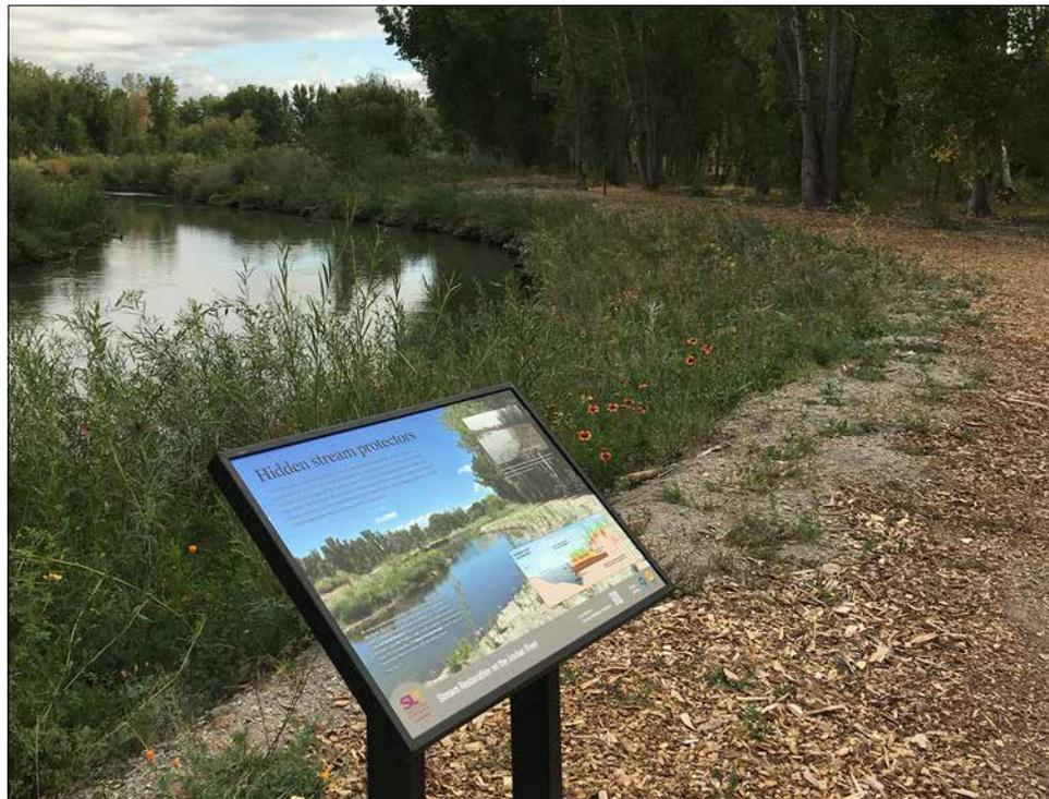
Once an aggressively eroding bank, native plants now thrive on this reconstructed streambank located at approx. 4850 S on the Jordan River. Deep roots stabilize the soils while stems and branches at the water's edge reduce floodwater energy.
