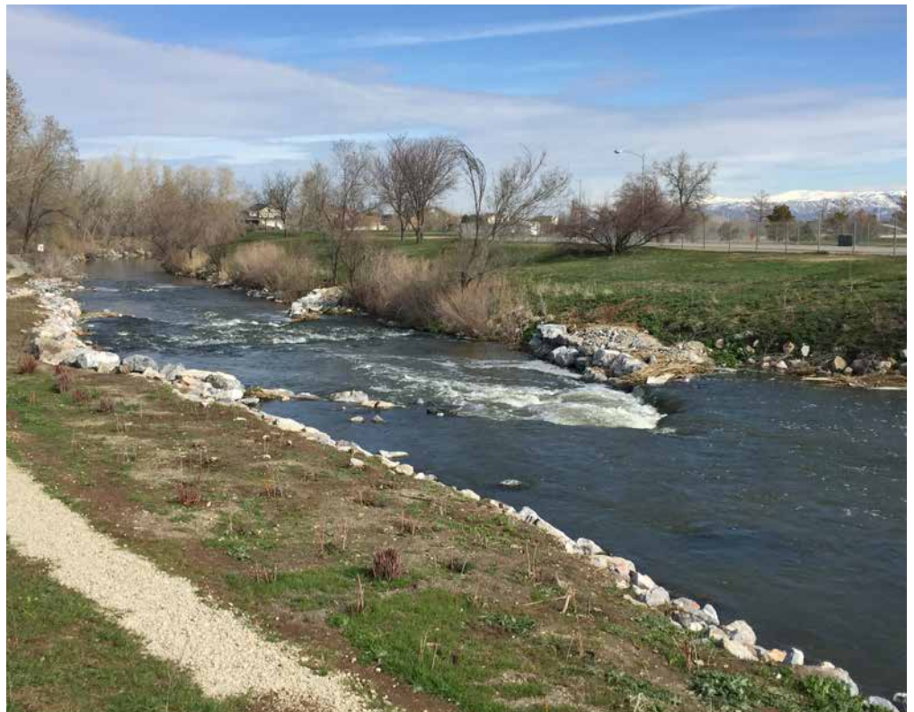
Newly designed stream channel at Winchester Park on the Jordan River
